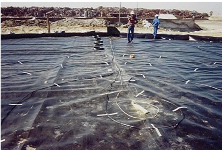
Figure 8: Cathodic protection system.
