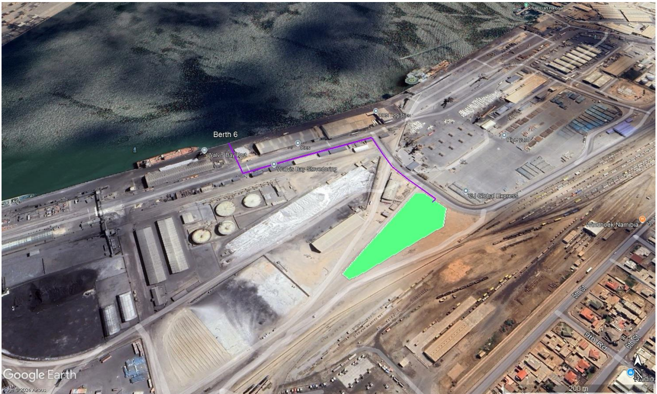
Figure 1: Sulphuric storage and handling facility (green) and pipeline (purple) from berth 6 to the facility in the Port of Walvis Bay. Please note: the four Rössing tanks are directly opposite from berth 6.
