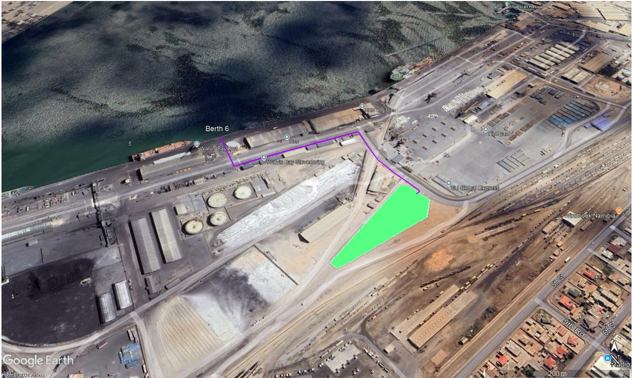
Figure 1: Sulphuric storage and handling facility (green) and pipeline (purple) from berth 6 to the facility in the Port of Walvis Bay. Please note: the four Rössing tanks are directly opposite from berth 6.
